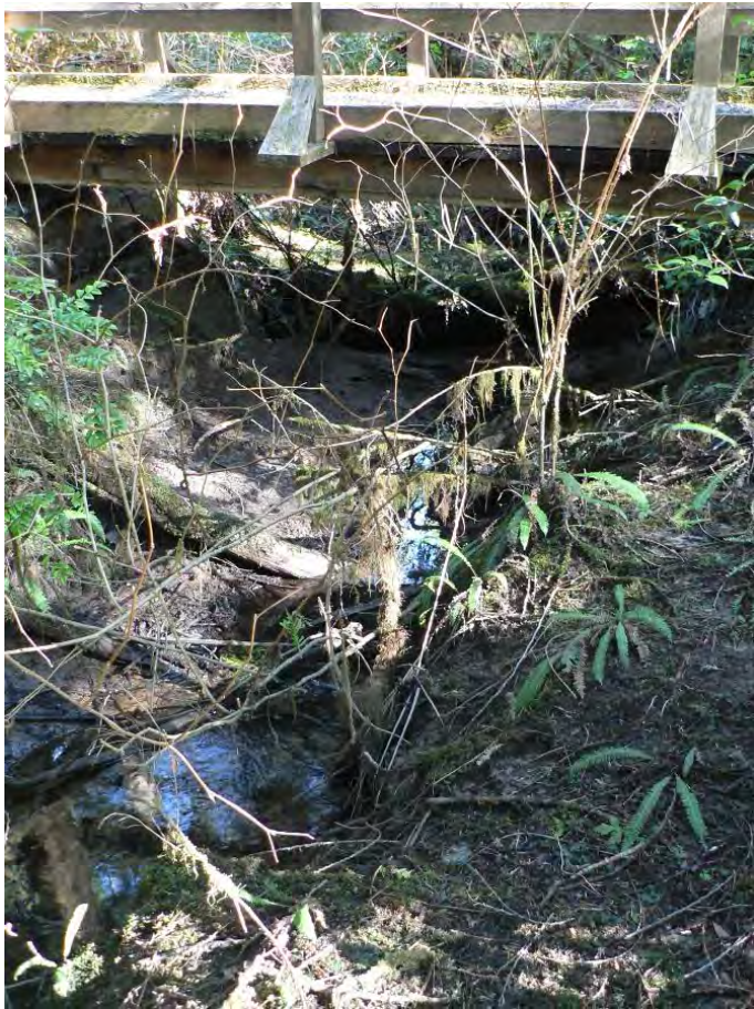
Photograph 1. March 5, 2019. View upstream on Stream #30 to footbridge crossing.
